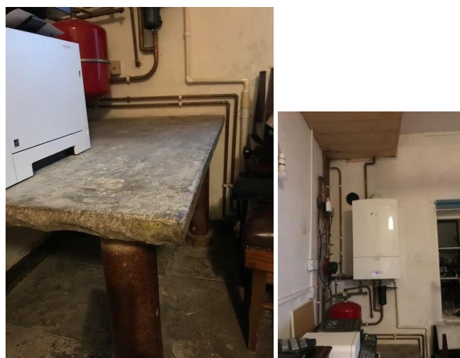
Photographs of salting slab and proposed approximate position internally of new vent (Source: Method Statement)
